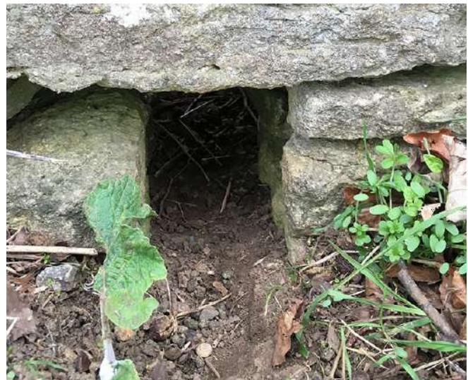
Figure 9: Hedgehog access in Cotswold Stone wall
