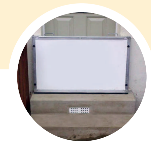
7. At Courtbrook 7 properties have been given flood-protection products. This includes door guards and airbrick covers.
