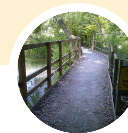
6. Near Dilly's Bridge the public footpath was raised. This reduces the flood risk to Courtbrook.
